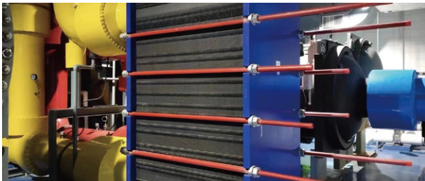
© Temperature-based control of plate heat exchanger
