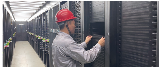
© Replacing missing blind flanges to avoid waste of refrigeration capacity
