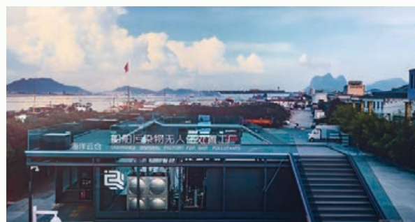
Marine cloud warehouse system for ship water pollutants prevention and control
