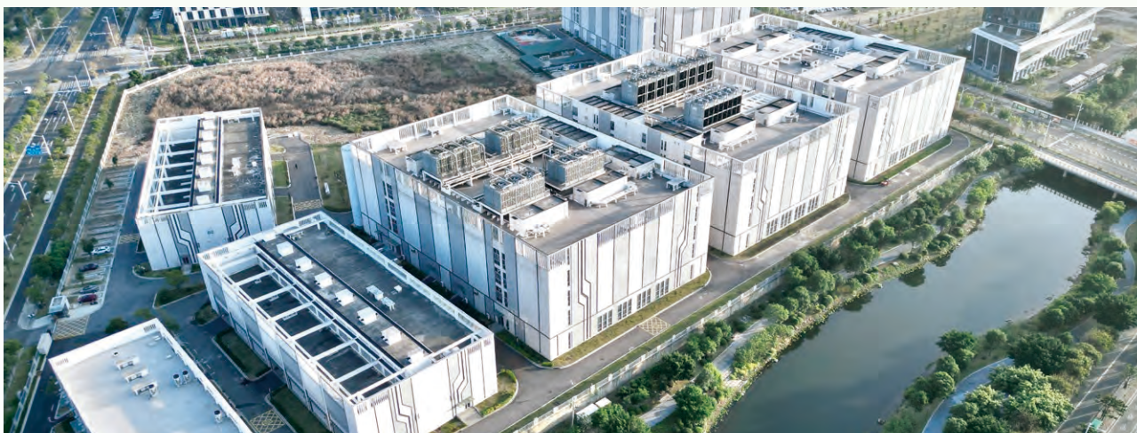
China Mobile (Fuzhou, Fujian) region level ultra-large data center.
