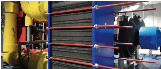
© Temperature-based control of plate heat exchanger
