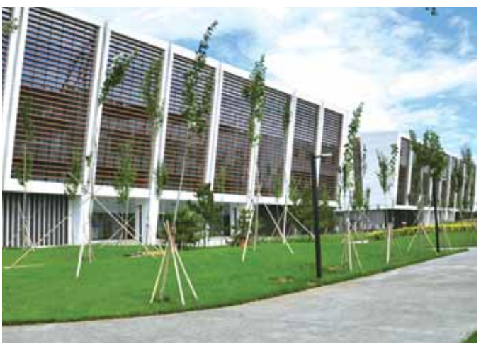
The first phase of data centre for China Mobile International Information Port
