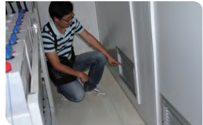
In Anhui, we launched partition cooling systems in our base stations
