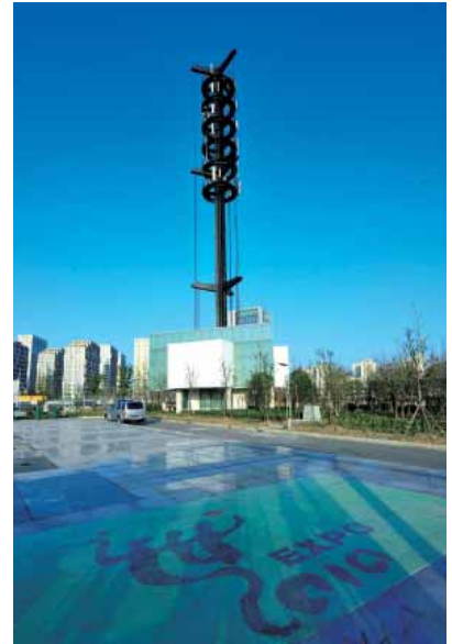
© A China Mobile base station in the Shanghai Expo Park
