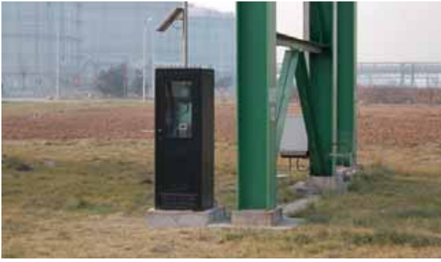
© In Hebei, we installed a waste water measurement monitoring equipment for a steel company
