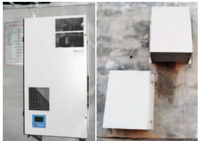
◎ In Hebei, we used an intelligent air exchange system in equipment rooms
