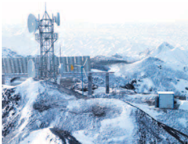
© In Xinjiang, we built base stations using alternative energy in remote areas
