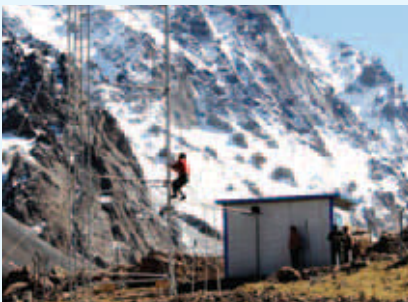
● In Xinjiang, we built base stations in the Tianshan Mountains
