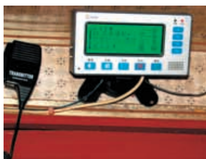
We installed mobile system safety control systems on fishing boats in Jiangsu
